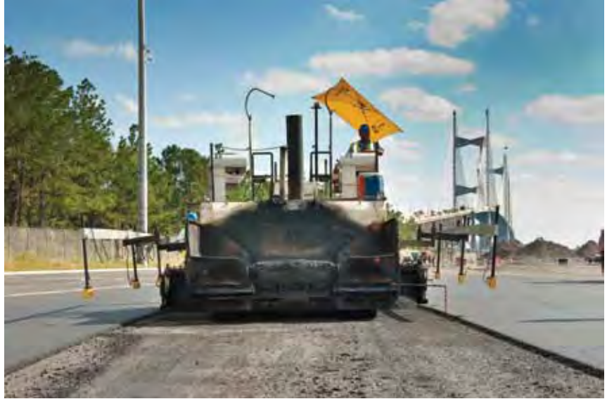
The Roadtec RP 185-10R paver was equipped with dual averaging skis and six Trimble ST200 sonic tracers (three on each side) to match asphalt slope requirements to the drain gates.
